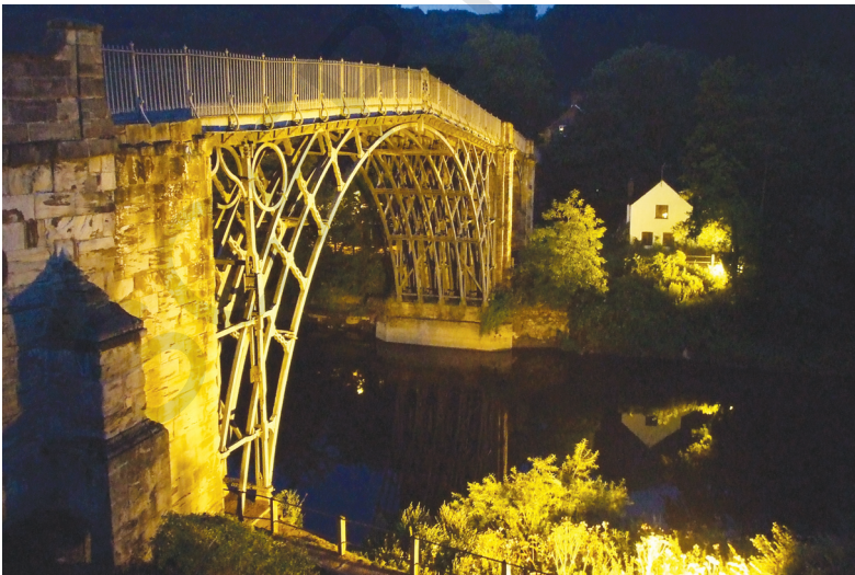
Fig. 14.2: The Cast Iron Bridge near Coalbrookdale, designed by the third Darby.
