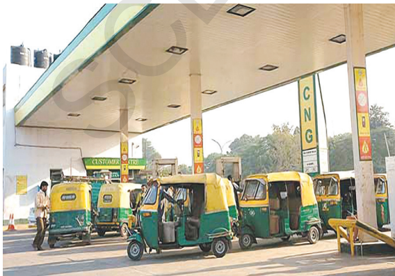
Fig - 3: CNG gas filling station
