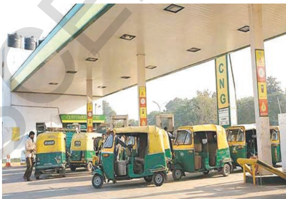
Fig - 3: CNG gas filling station
