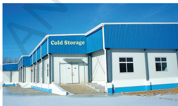
Fig-28 Cold storage unit
