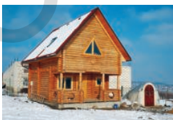
This house is built with wood. We can find it in earth quake zones.
