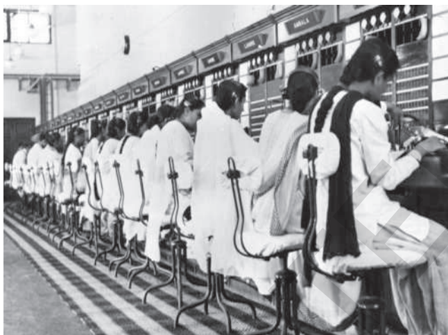
Fig 18.6 : Operators at work in the New Delhi Telephone Exchange - 1950's
