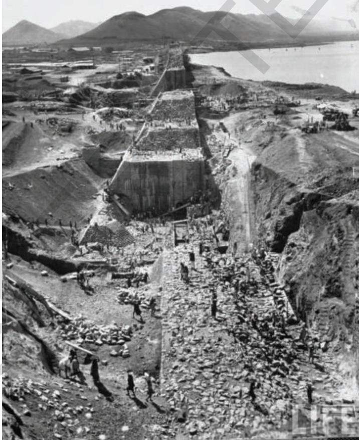
Fig 5.1 : Tungabhadra Dam Construction - 1952
