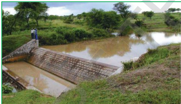
fig-1: Communitybased masonry dam
