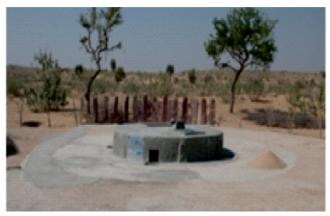
Fig. 8.10: Taanka with Aagor (upper part is covered with platform of stones or other available material)
