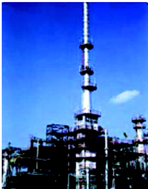
Fig. 5.5: A petroleum refinery
