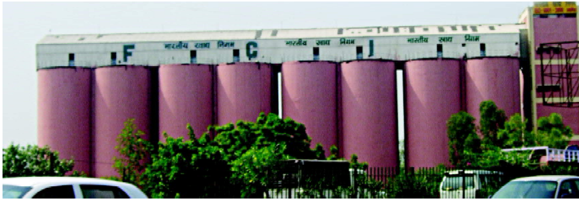
Fig. 1.10 (a) : Silos for storage of grains
