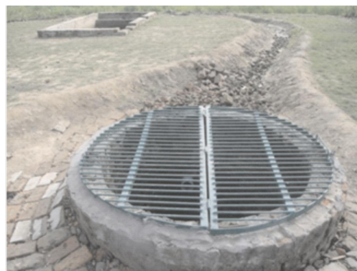
Groundwater recharge through abandoned well
