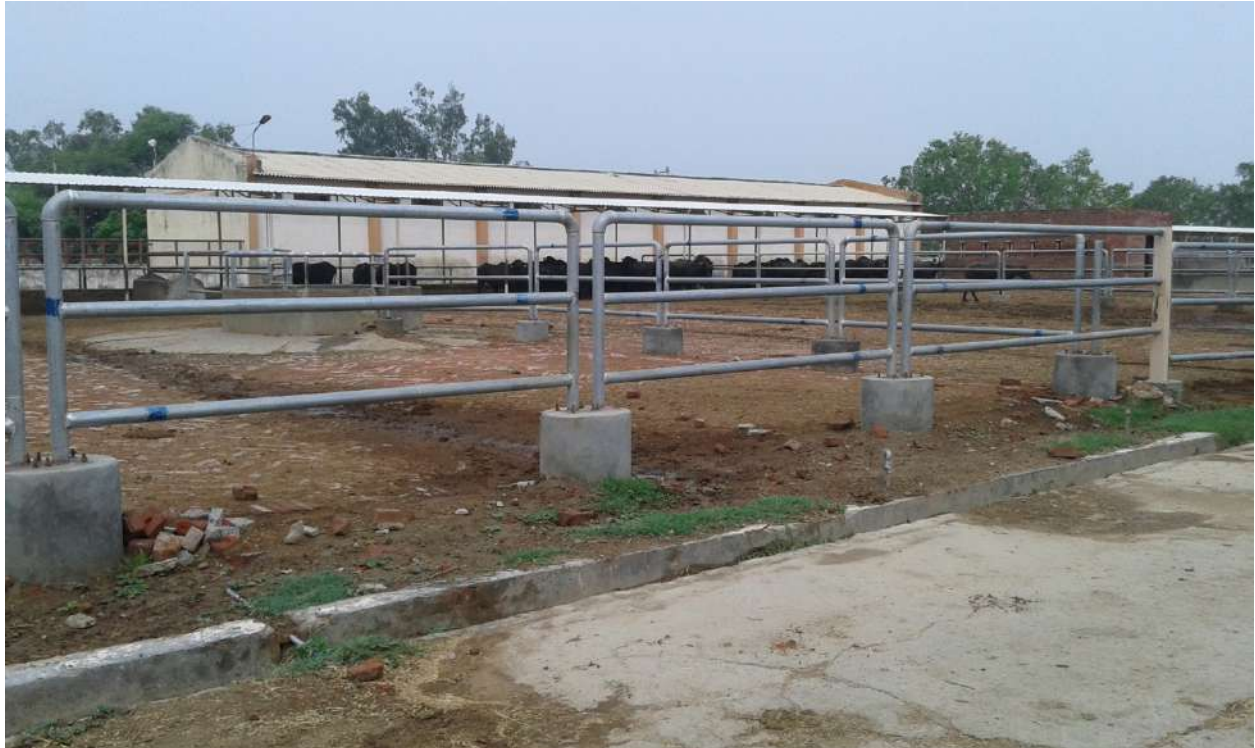
Photograph 4.3: Another view of loose house
