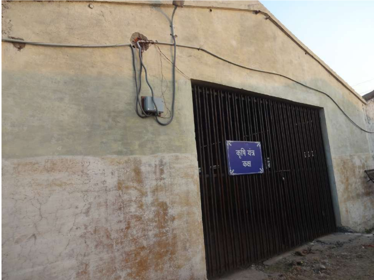
Photograph 4.17: Photograph of implement shed
