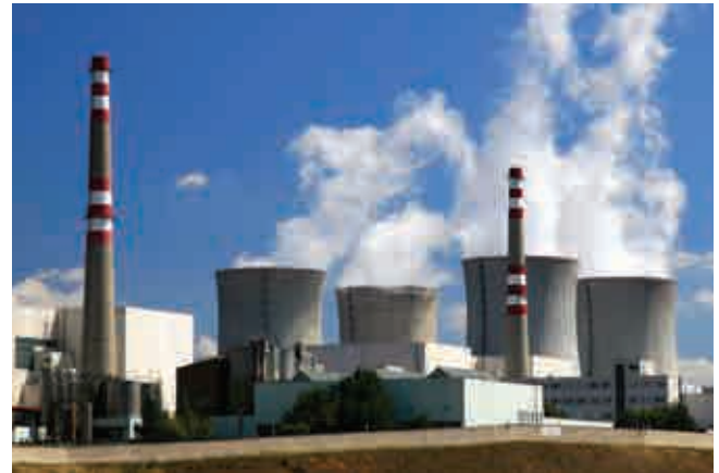
Figure 9.17 : An Atomic Power Generation Plant
