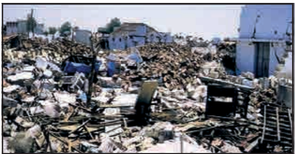
Figure 5.2 :The Bhuj earthquake 26 th January,2001
