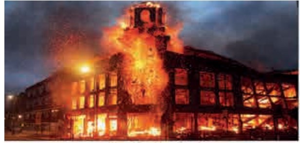
Figure 5.8 : Fire Incident (Source : http://google.com )
