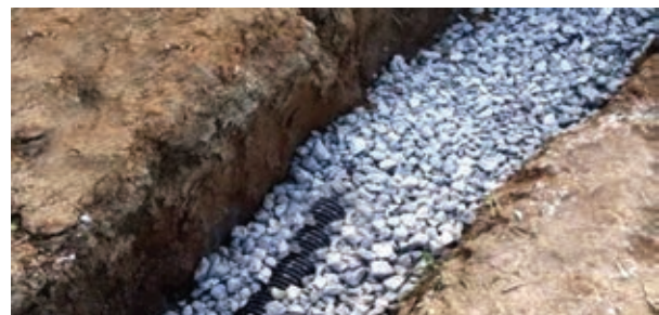
Fig 7.11 : Tile drainage
