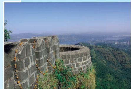
Figure 1.13 : Khadakwasla Dam as seen from Sinhagad
