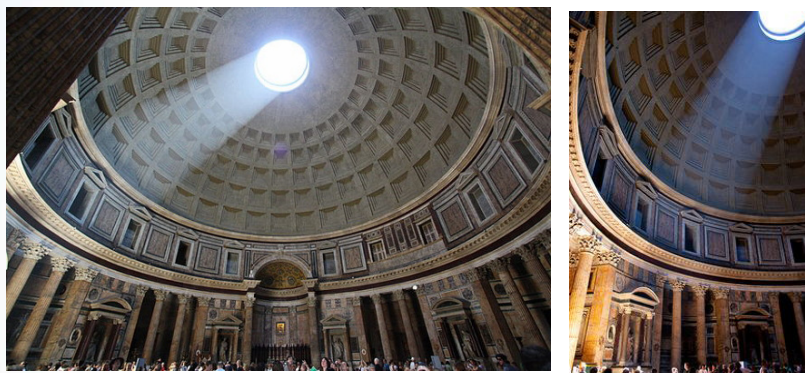
Cupola - a dome rising over the roof of a building – achieved by rotating an arch on its axis.
