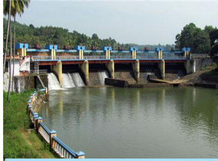
Fig. 8.8 : A flood gate in Aruvikkara-Kerala
