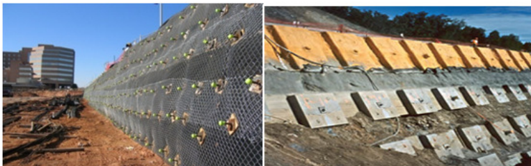
Fig. 8.12 :Rock bolts to prevent slope failure
