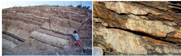
Fig. 4.22: Examples of faults
