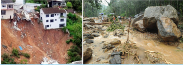
Fig. 8.10: Effects of landslides
