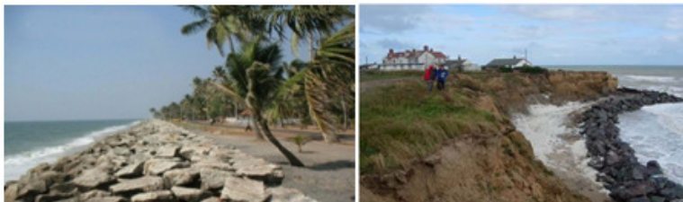
Fig.8.17: Sea walls built for coastal protection
