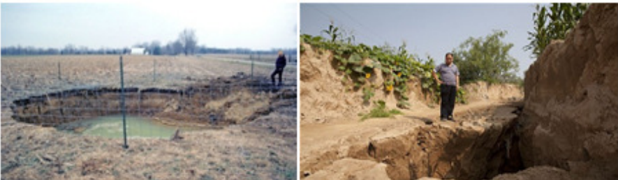
Fig. 6.5: Land subsidence due to mining
