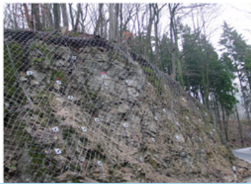
Fig.8.11: A slope covered with wiremesh
