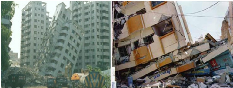
Fig 8.3 : Collapse of buildings during the event of earthquakes
