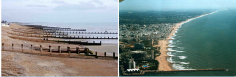
Fig.8. 18: Groins built for trapping long shore currents
