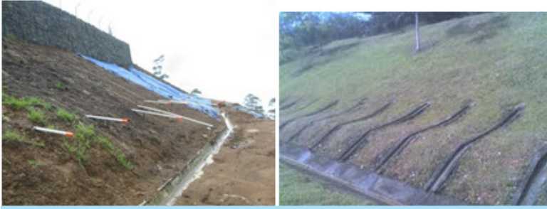
Fig. 8.13: Drainage pipes along slopes.
