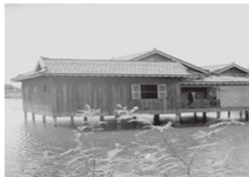
Fig.8.9: A house constructed in flood zone.
