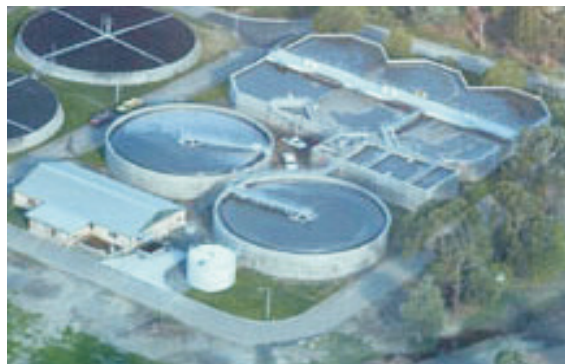
Figure 10.7 An aerial view of a sewage plant
