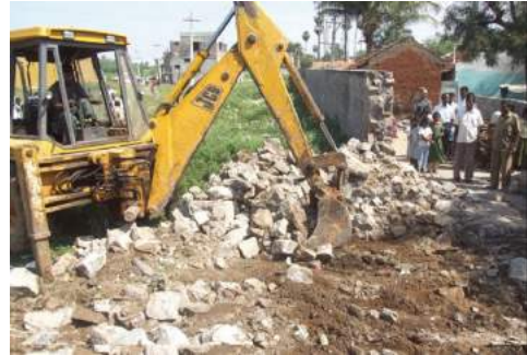
Picture 6.1 Demolition of untouchability wall
