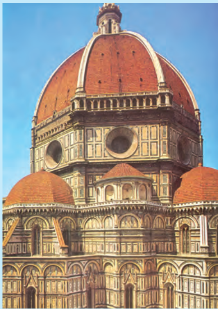
The Duomo, the dome of Florence cathedral designed by Brunelleschi.
