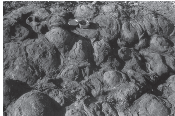
Fig.6.4 : Exfoliation (Flaking) and granular disintegration
