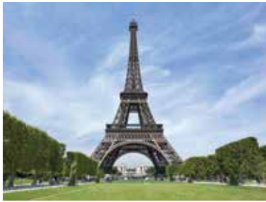
Eiffel Tower: France
