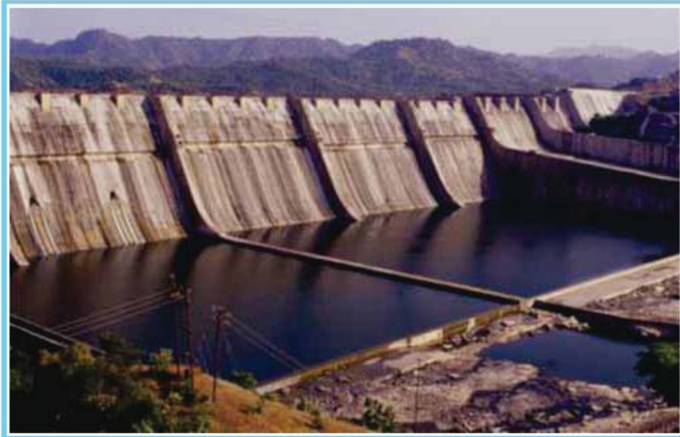
Fig : 18.4 Sardar Sarovar Dam
