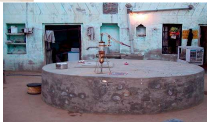
Figure 2.30: Small cylindrical underground well (tanka)
