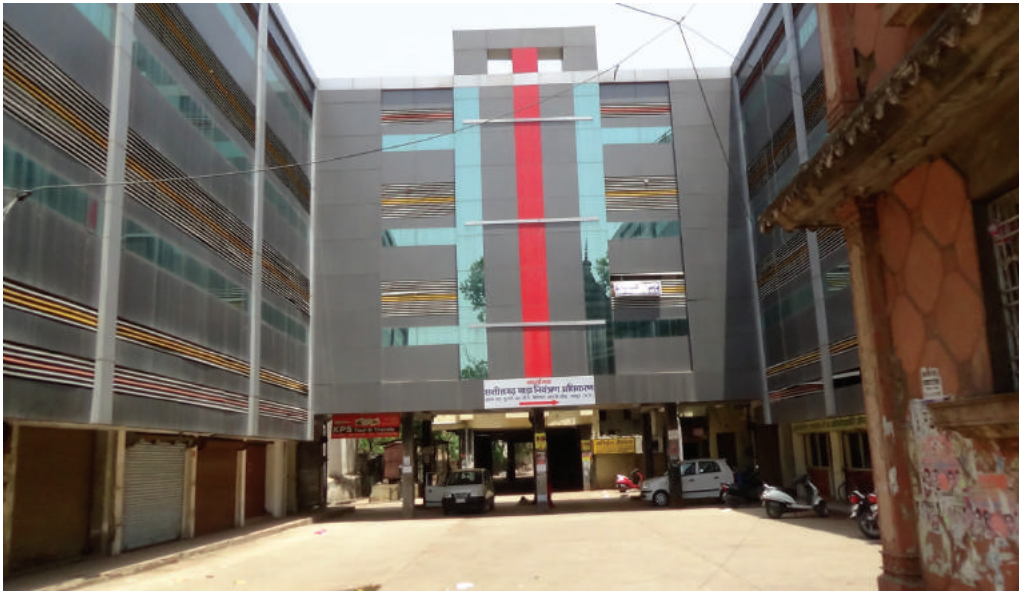
Figure 18.8: An office building
