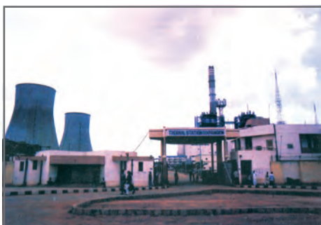
Fig 3.10: A view of a Thermal Power Station
