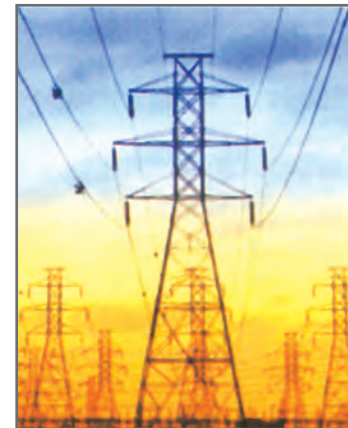
Fig. 3.7: National Power Grid to supply Electricity
