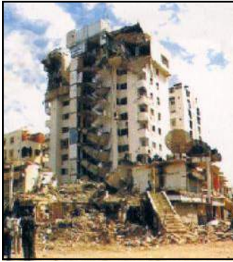
Fig. 3.3a: Destruction caused by an Earthquake in Gujarat
