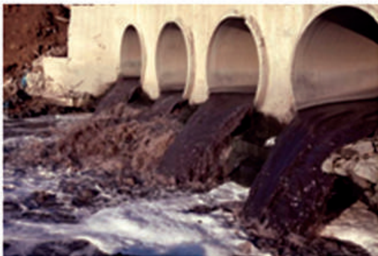
Figure 1.5 Sewage water in cities
