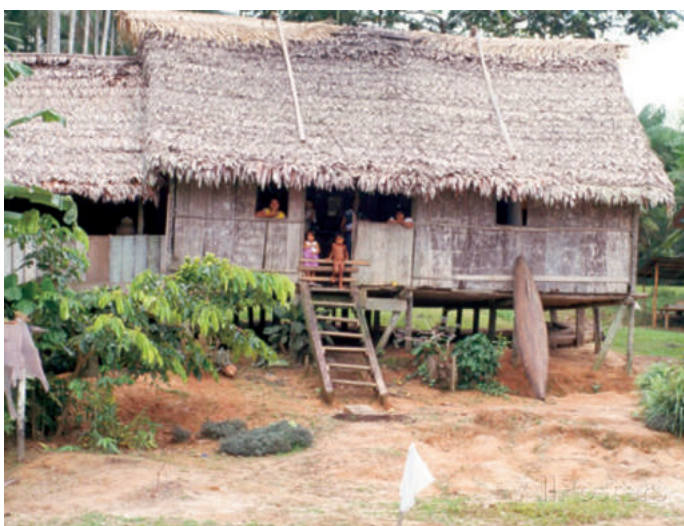
Fig. 6.1: House of Amezaan Besin
